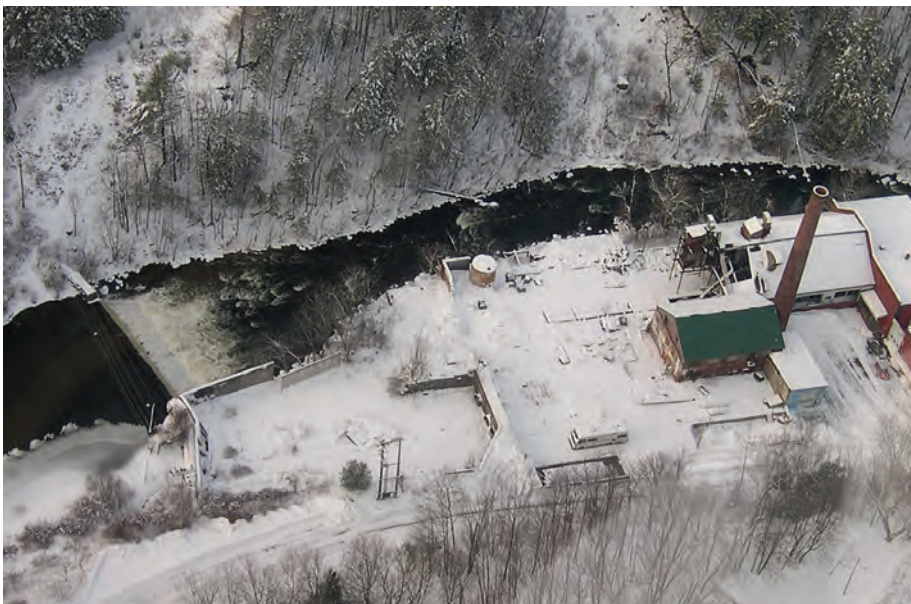
Gardiner Paperboard Dam, Winter
